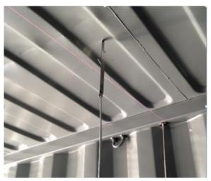
NEED TO REPAIR UNDERTERMINED If upward dent is more than 100 mm (4 in) above the lower face of the top side rails, repair is required.
